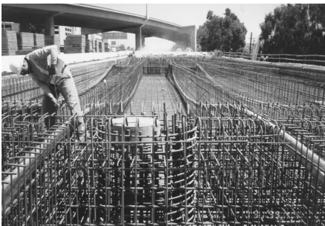
Figure 1: A post-tensioned box-girder bridge under construction
